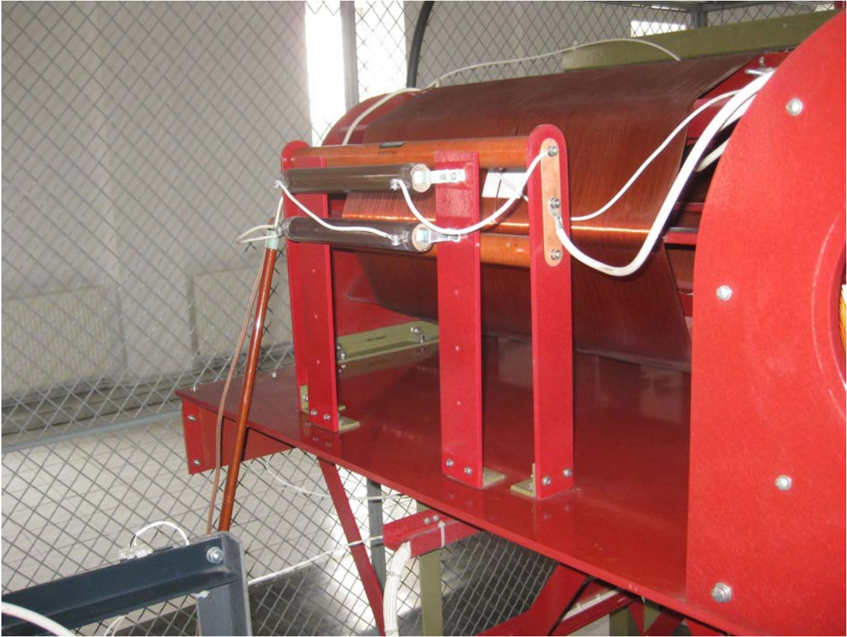
Figure 7. Cable Installation - Right Side.
